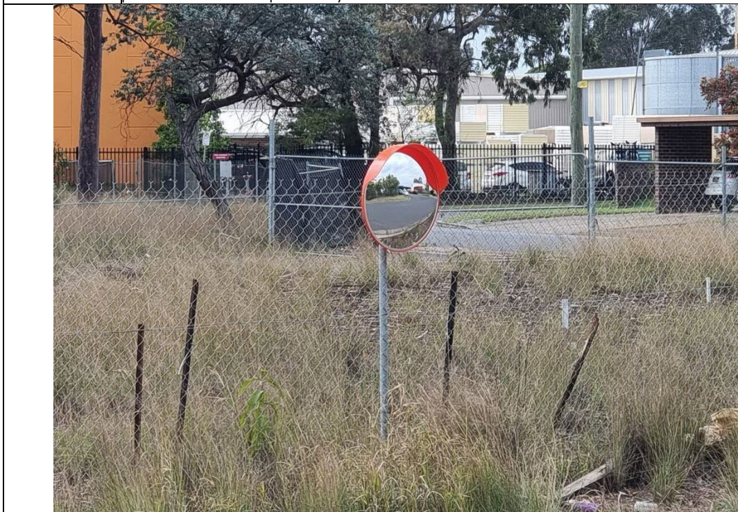
Photo 3 Dunheved Circuit, opposite main site entrance, showing convex mirror as traffic as required by CoA B2.
