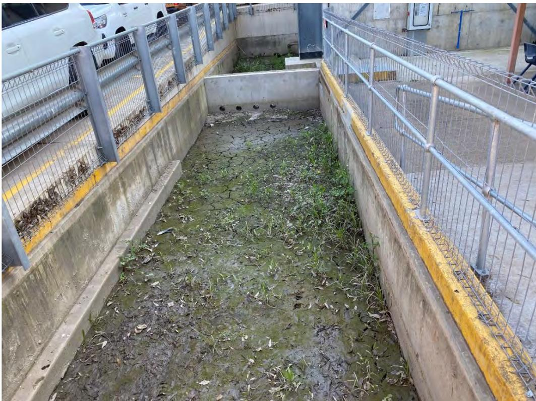
**Plate 18 - Stormwater sandfilter system**
