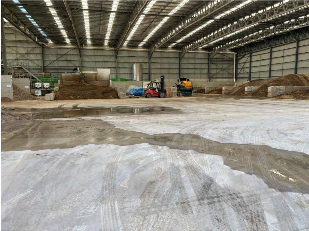
**Plate 11 – Clean workshop floor showing appropriately banded storage areas for stockpiles**
